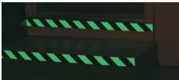
Photoluminescent area marking
