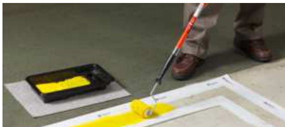
Paintstripe & floor marking area
